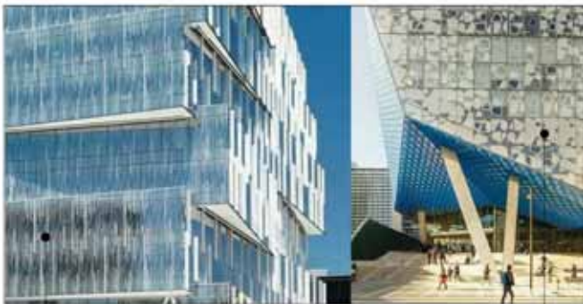
DOUBLED GLAZING WITH FRITTED PATTERN (PATTERN TO BE DEVELOPED)
