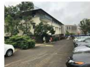
2. VIEW OF CARPAK AND WEST ELEVATION
