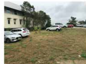
3. VIEW OF NEPEAN HOSPITAL FROM NORTHERN CARPAK
